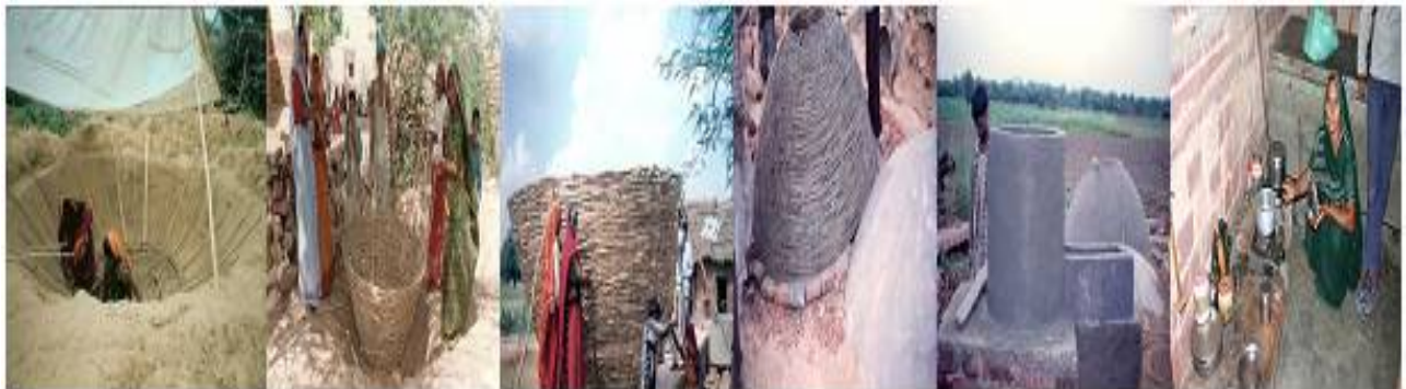
PHOTOS-8 (A) TO (F): TRAINING ON THE STEP-BY-STEP CONSTRUCTION CUM BIOGAS UTILISATION OF CUM-DEMO GRAMEEN BANDHU BIOGAS PLANT (GBP) OF EVD STAFF, REEVOCS AND VILLAGERS BY INSEDA. THE POOR LANDLESS VILLAGES WOMEN TRAINED GET WAGES SITTING IN THEIR VILLAGES AT THEIR SPARE TIME, AS AND WHEN THE WEAVING OF BAMBOO STRUCTURE ARE BUILT IN THE EVD AS WELL AS OTTHER VILLAGES BY WAFD TECHNICIANS
