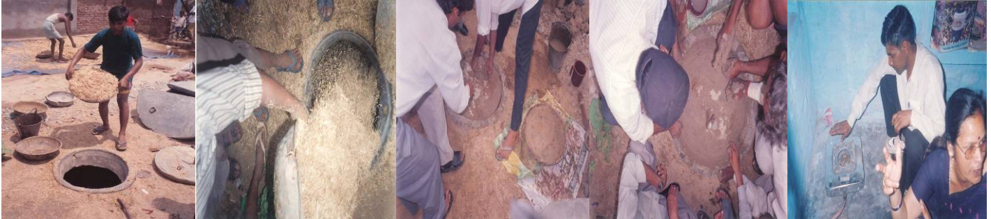
PHOTOS-6 (A) TO (E): BIOMASS EXPERIMENTAL BIOGAS PLANTS (IT IS IN OPERATION SINCE 2003, WITH MUSTARD HUSK, AS FEEDSTOCK, WHICH IS AVAILABLE IN ABUNDANCE DURING THE HARVESTING SEASON.
