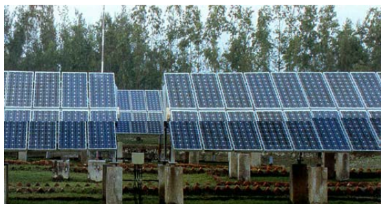
A view of a stand-alone solar photovoltaic array for generation of electricity
