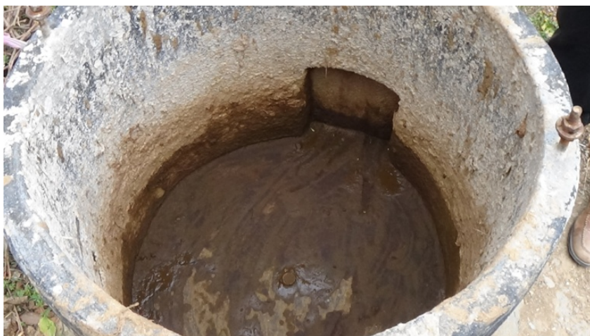
The slurry mixing tank of the biogas plant
