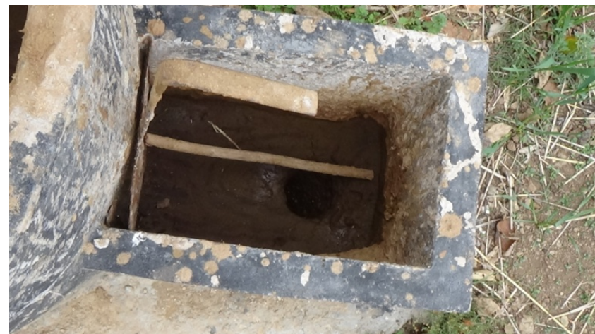
The inlet of the biogas plant
