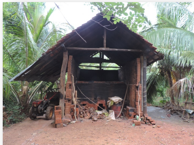
Fig 5.3.2 Dharmaratne's improved and permanent brick kiln
