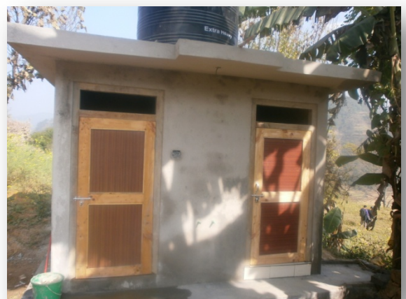
Fig 5.4.3 Toilet and water tank built after Hydram installation
