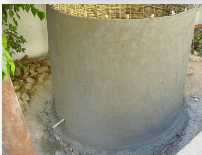
Fig 5.2.6.1 and Fig. 5.2.6.2 Bamboo-cement based rain water storage tank under construction
