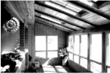
A sunspace or attached greenhouse relies primarily on convection to move heat from the sunny space to other adjacent rooms.
